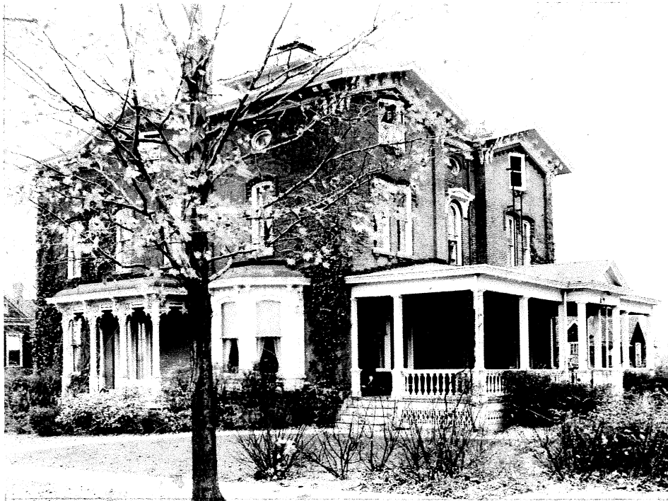
The Delta Upsilon House, 1938. The front steps and railings, shown above, have been replaced with a porch. The original, exterior dark green trim was painted white in 1937, enhancing the Victorian architecture.
